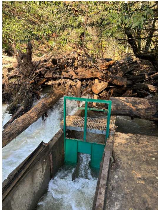
The Fall Creek fish ladder plugged with debris was preventing fish passage in the Coos watershed.
